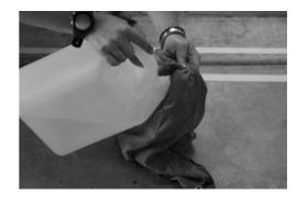
Apply the adhesive to the floor between the lines, in either straight or zigzag lines.
